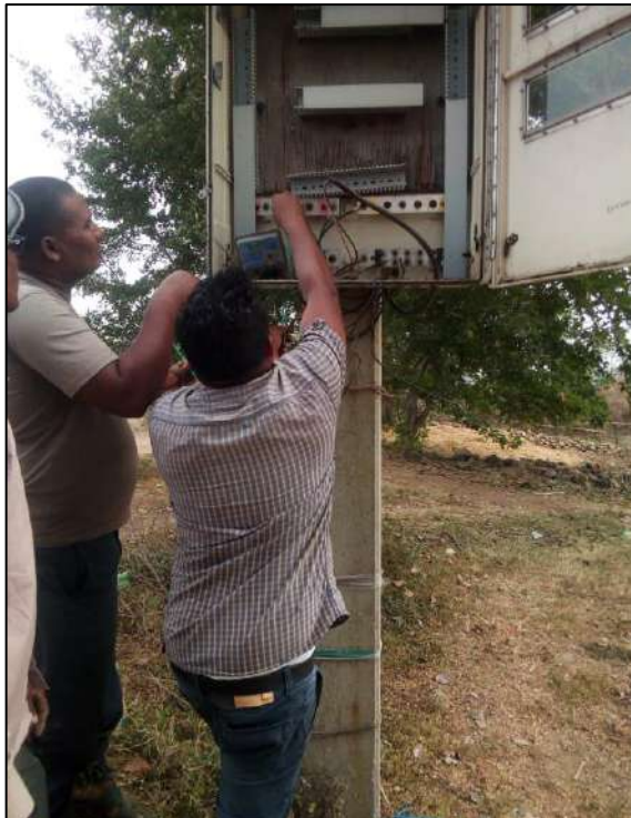
Repairing work of starter Panel of Submersible Pump (3HP) Near Muktidham & Sanjay Nagar – Nariyara
