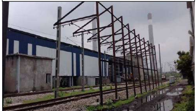
Water Sprinkler arrangements at Wagon tripler site
