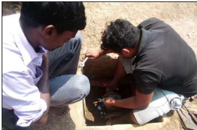
Repairing of Gate valve on Overhead water tank – Nariyara and Rogda
